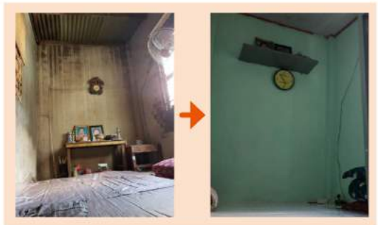
Before and after the repair work
