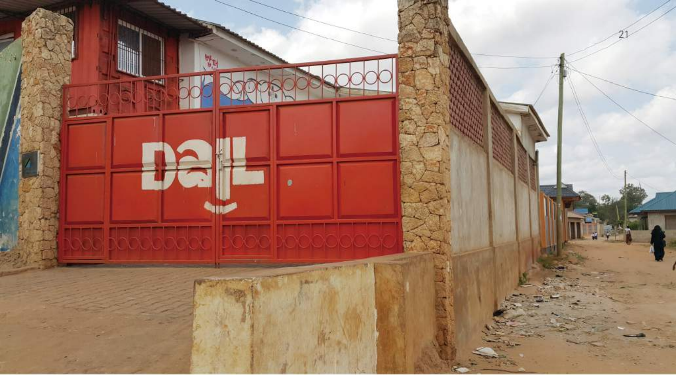
The wall on the right side of the center where a sidewalk and a rain shield will be installed
