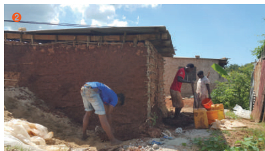
① Photograph of construction of house for Sophia
