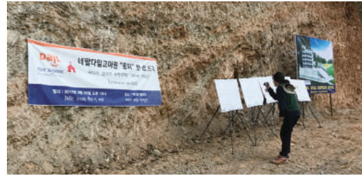
Displaying the floor plans and drawings of the orphanage after sculpting the hillside with fork crane
